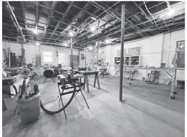
The basement (aka, future maker's space)
